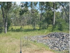
Drain condition and rock armouring IPEE southern sediment pond outlet
