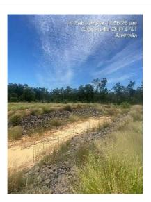
Drain condition and rock armouring IPEE southern sediment pond outlet – 2
