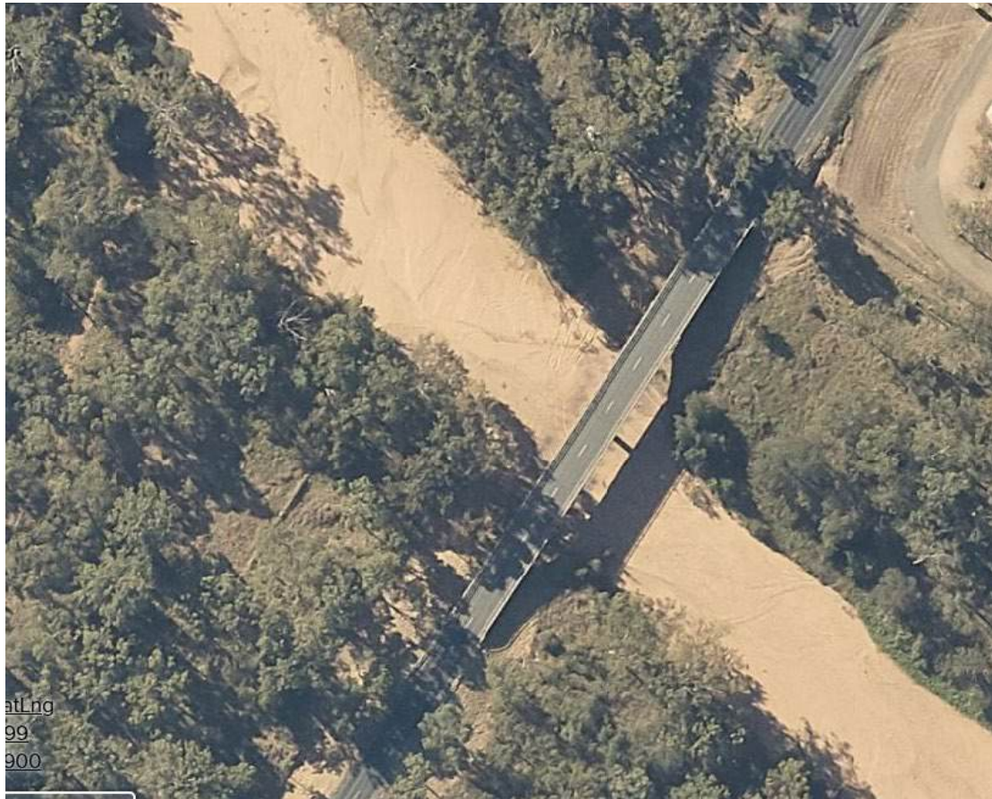
Figure 4.8 – Existing Peaks Downs Highway Bridge over the Isaac River
