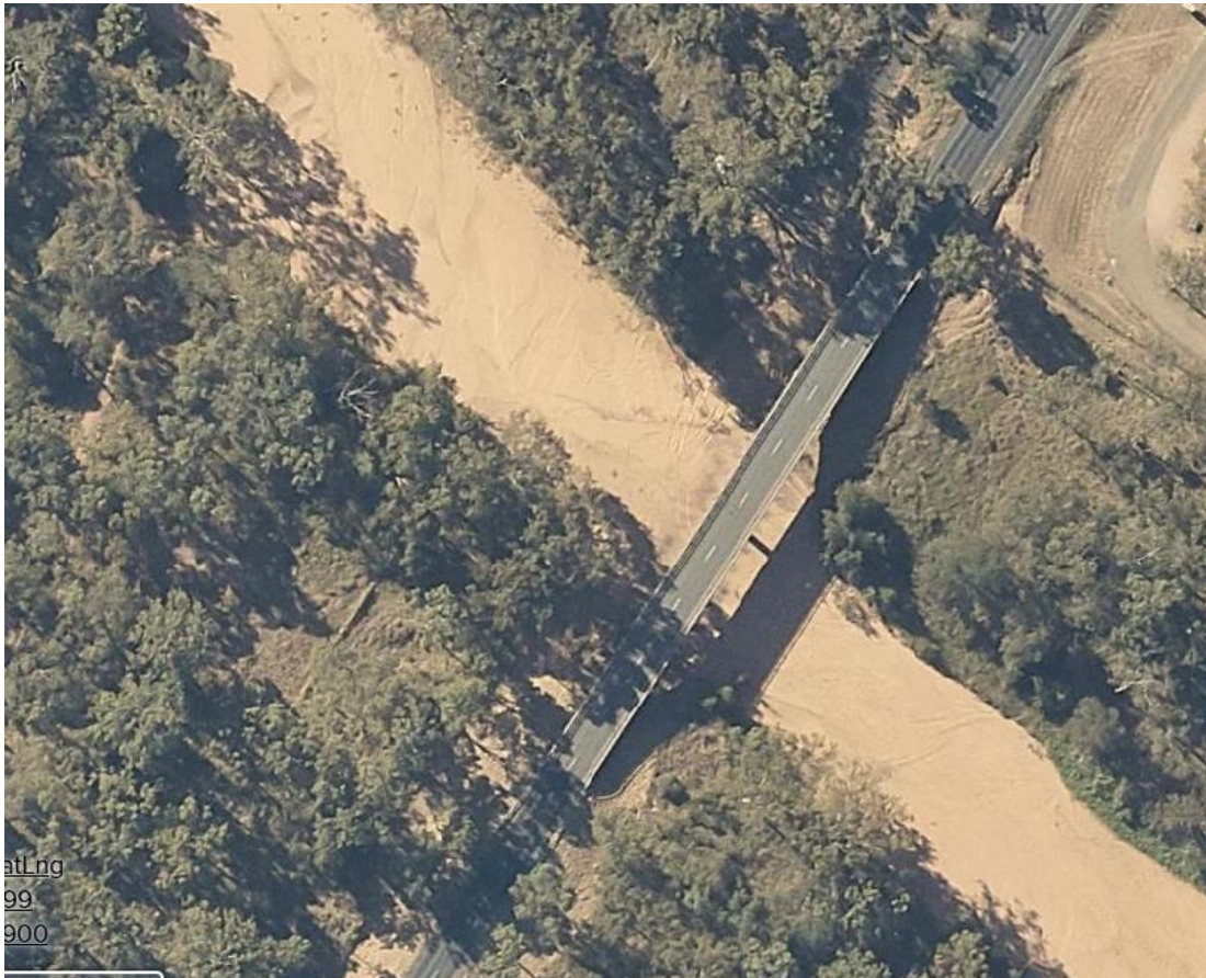
Figure 7-5. Existing Isaac River bridge crossing on the Peak Downs Highway.
