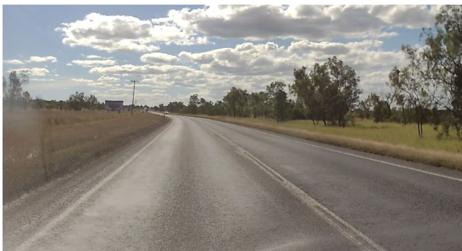
Figure 4.3: Moranbah Access Road
