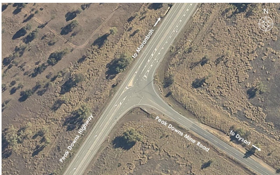
Figure 4.12: Peak Downs Highway and Peak Downs Mine Road Intersection
