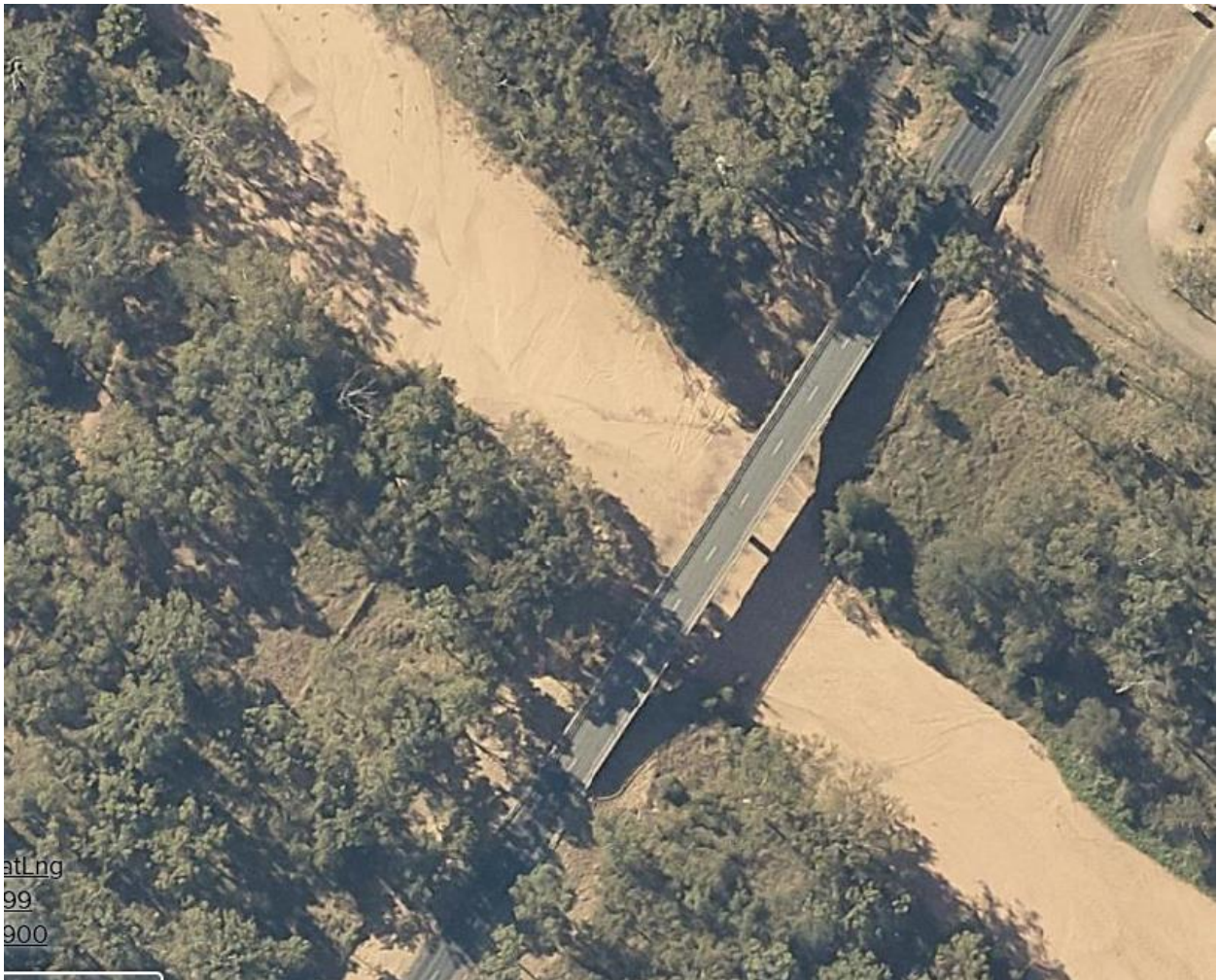
Figure 23-4 Existing Peaks Downs Highway Bridge over the Isaac River
