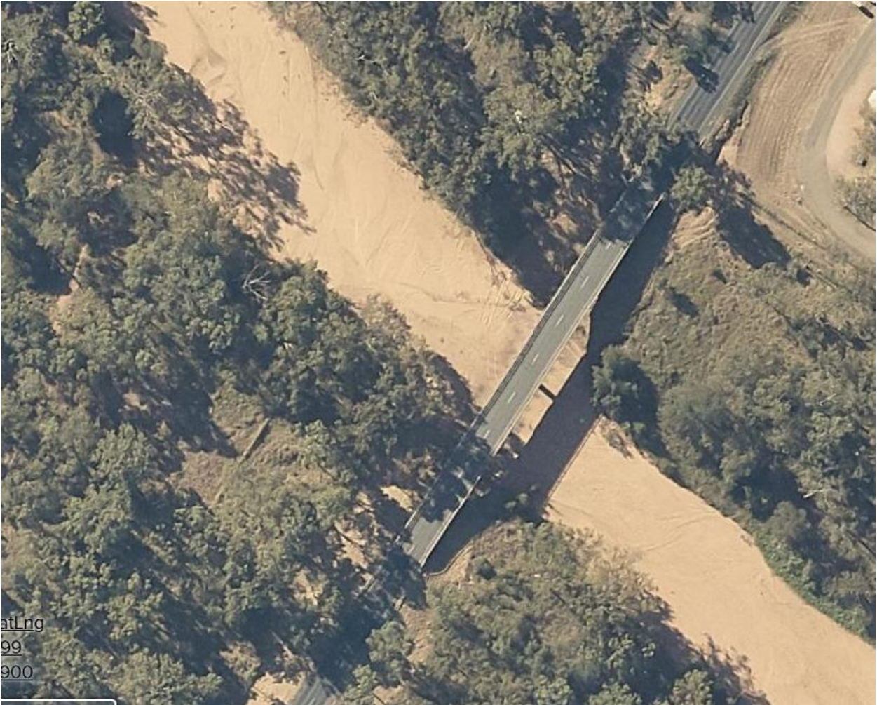
Figure 4-33 Existing Peaks Downs Highway Bridge over the Isaac River
